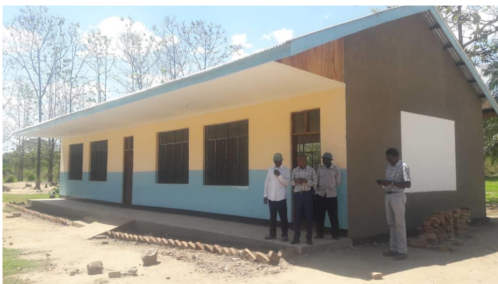
Figure 12: Idete primary school classroom built by KVTC social fund project. 29 th Oct 2019.
