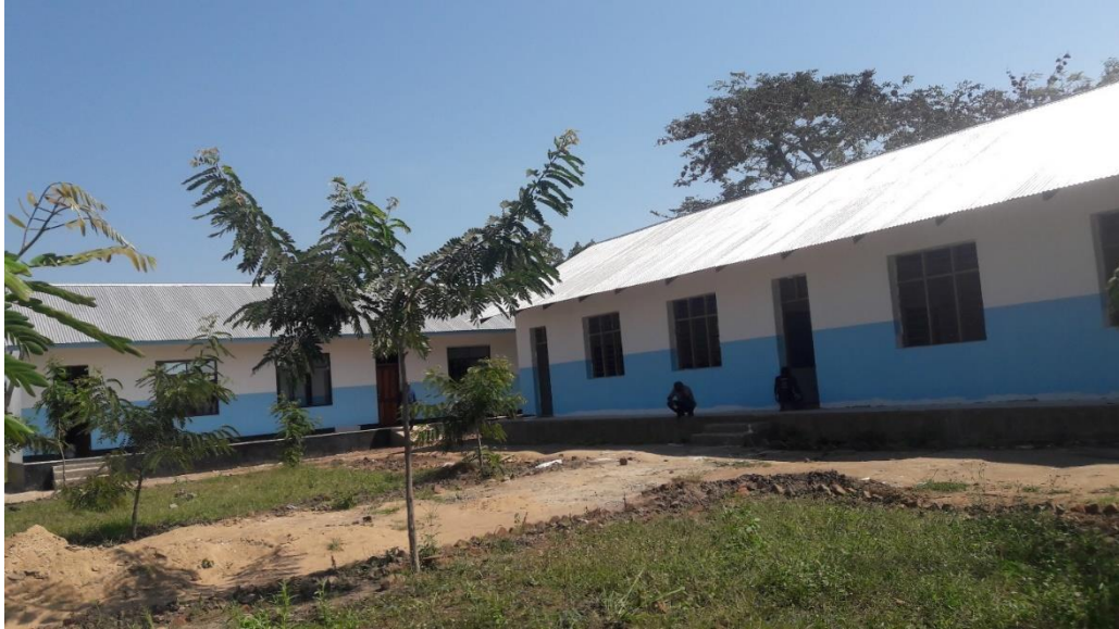
Figure 11: Ulanga Secondary school> Built with funding from the Community, Government, Selous and KVTC Social Fund
