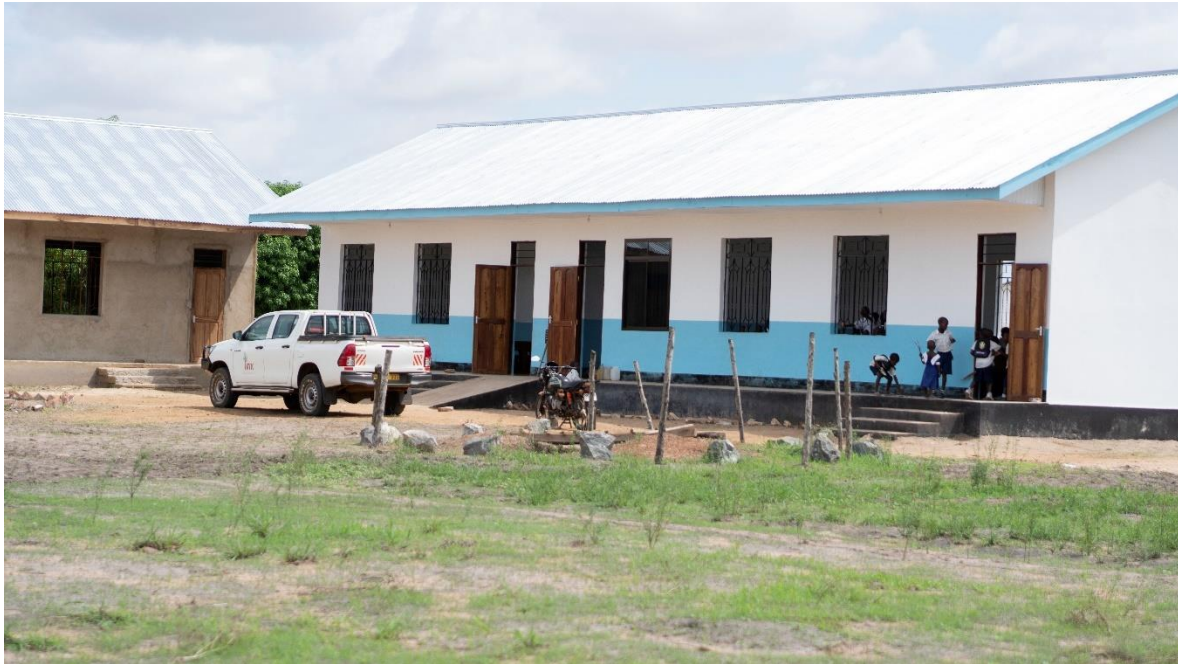
Figure 11: New Mavimba “B” primary school built with funding from the Community, Government, and KVTC Social Fund
