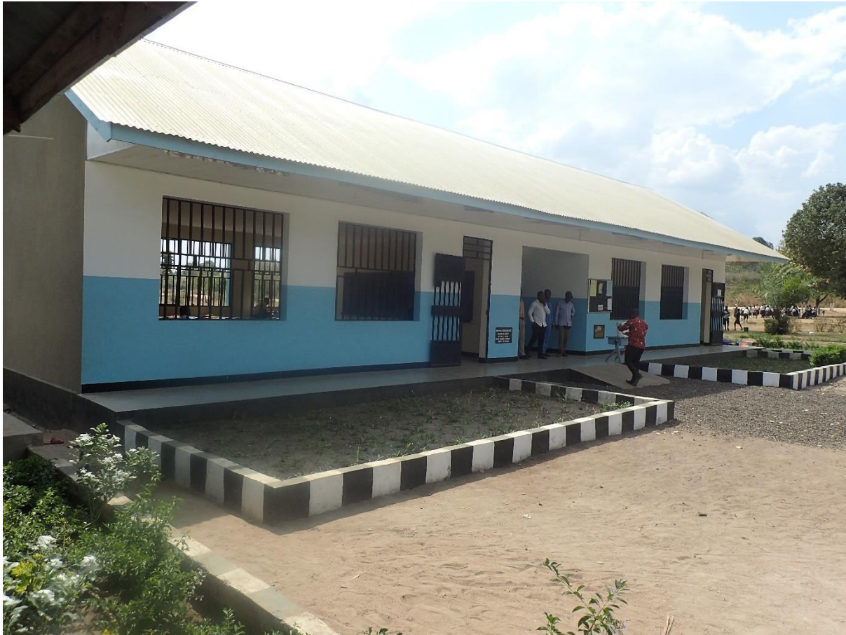
Figure 11: Idete Crossing Primary School Double classroom and Head Teacher Office built with funding from the Community, Government, and KVTC Social Fund.
