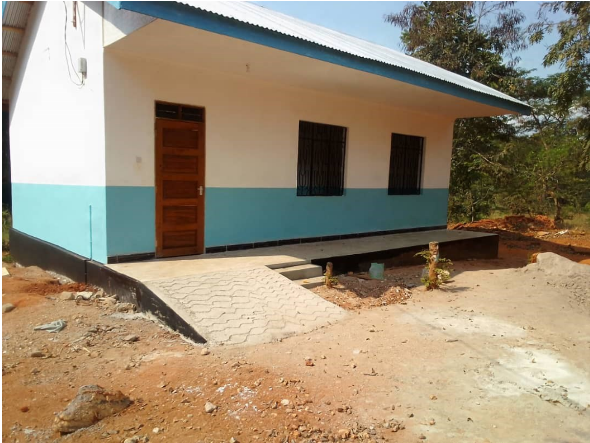
Figure 12: Ikungua Primary School single classroom built with funding from the Community, Government, and KVTC Social Fund.
